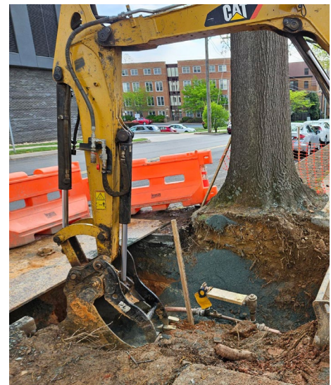
Left: Aerial showing location of Garrett Street tree removal; Right: Utility trenching immediately adjacent to tree forcing its removal (Image source: Steven Gaines)
