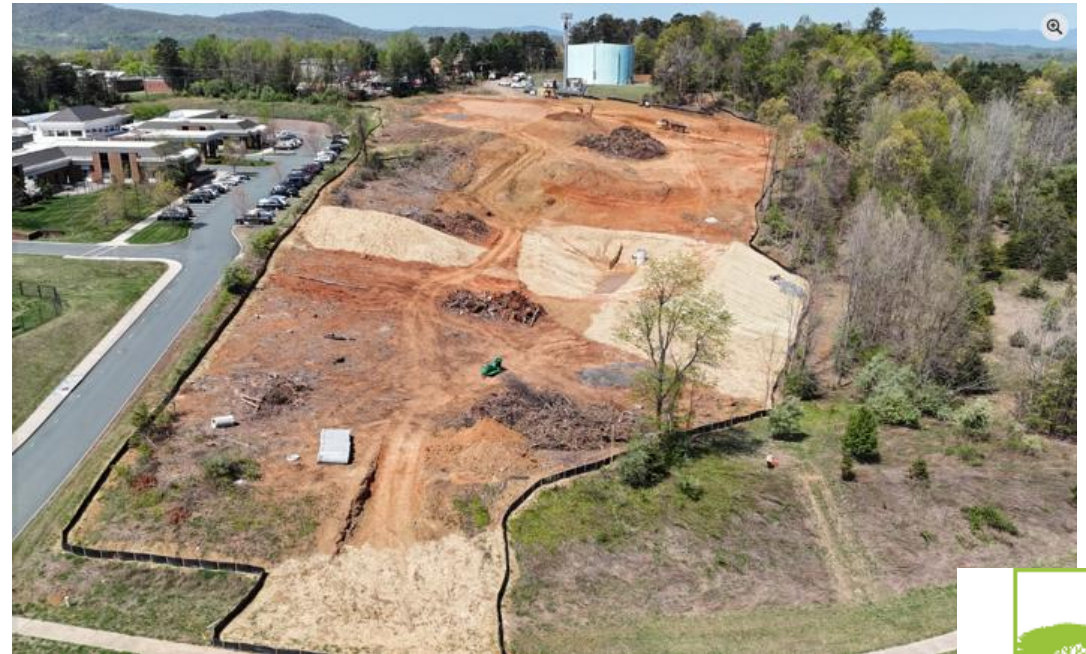
Albemarle County Service Authority Avon Operations Center And American Tower Property
